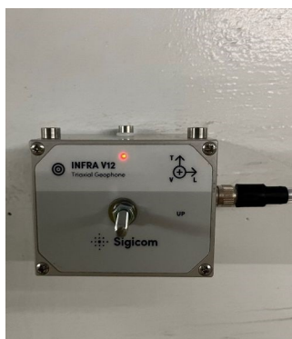
INFRA V12 monitoring vibration
