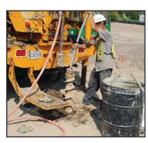
2. Drill the borehole and slide the borehole geophone into place.
